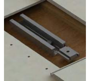
5. Slide the supplied channel strut through the Tile Strut.
