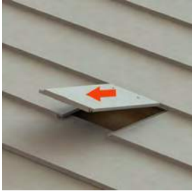
1. Remove the tile and locate the rafter.
